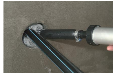
Filling the annular gap
