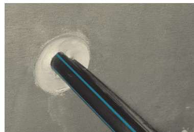
Smooth off excess sealant
